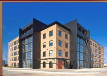
Finished Building - Front
